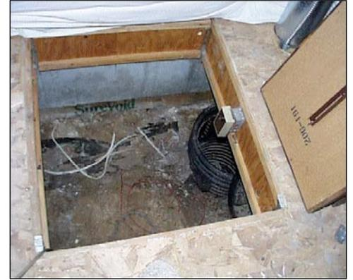
Some crawl spaces have humidity and temperature sensors that turn ventilation fans on and off. Do not set the humidity sensor above 40% relative humidity (RH) or the thermostat below 40°F.
