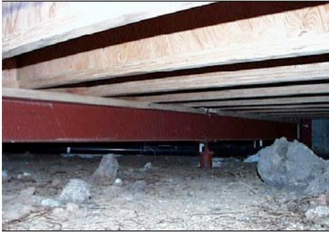
A ground cover (10 mil plastic sheeting or equivalent puncture- and moisture-resistant material) can help control a moisture problem in your crawl space. It is best for the ground cover (also called “vapor retarder”) to be completely sealed to the
